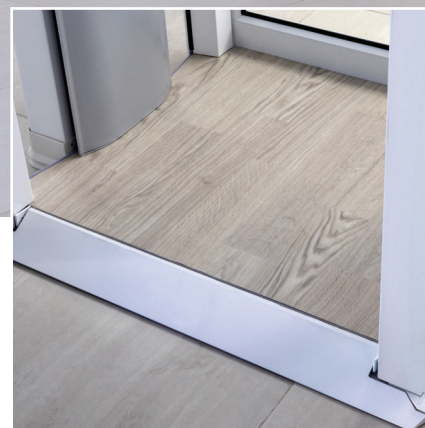
Sloped threshold and attractive non-skid flooring
