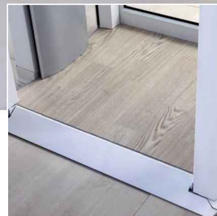
Sloped threshold and attractive non-skid flooring
