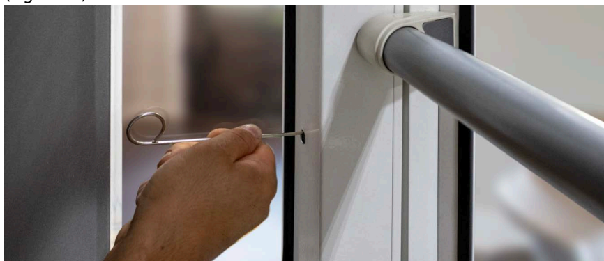
Figure 11: Inside access to emergency opening
